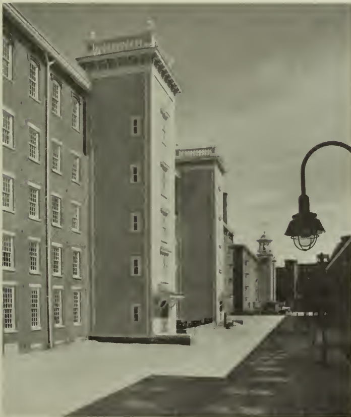
Figure 9. The window solution represents an important advance in the way in which aluminum windows can be designed to capture more fully the appearance of historic windows in larger buildings. Right photo shows wood sash in bottom row and aluminum in the upper three rows. Photos: Jim Higgins ©
